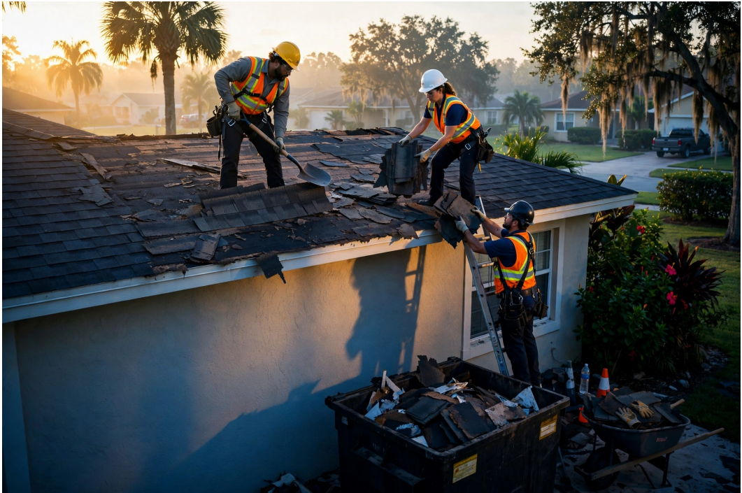
Figure 5.3: Fourteen field employees start every Delgado job. Burden is priced before the first shingle moves.
